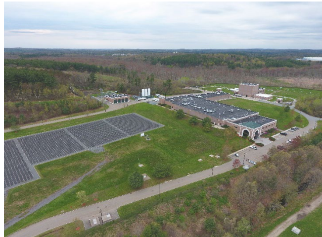
Carroll Water Treatment Plant
